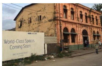
Figure 2, Castle hotel standing next to the debris of demolished Java Lane houses. (Source: Thushni De Silva)
